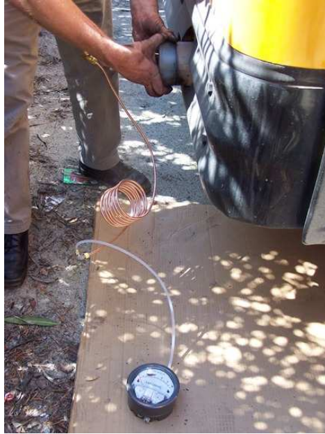
Photograph 4.2.4.1.1 Back pressure method to evaluate exhaust system leaks using a silicon stopper and magnehelic.
